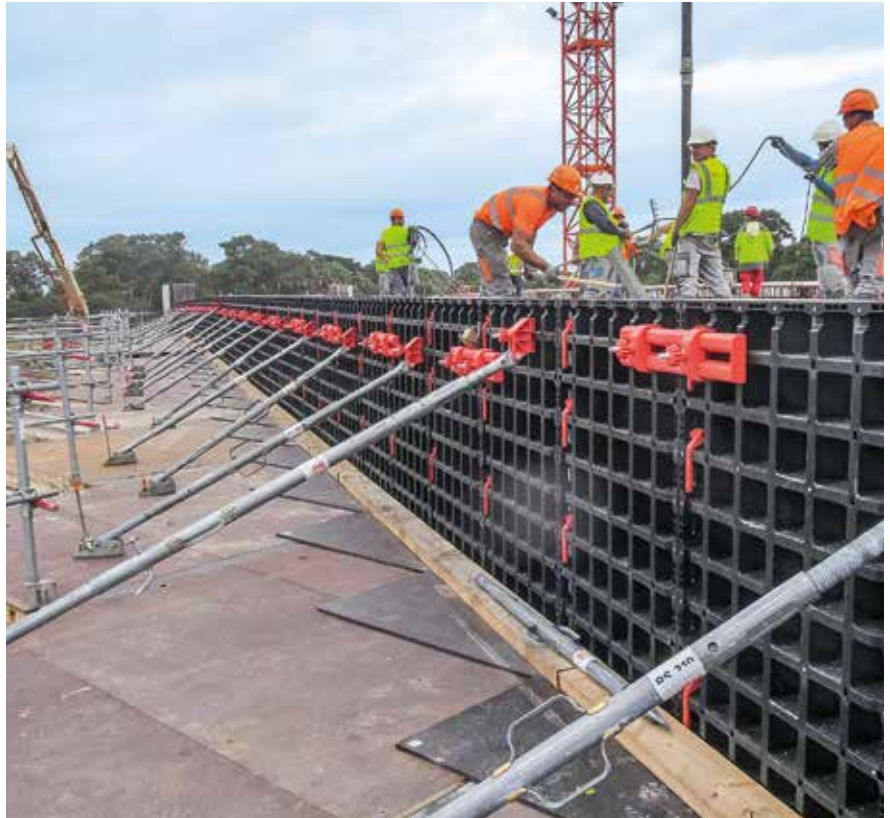
With its small panel sizes and ease of use, DUO is the ideal system for forming foundations.
