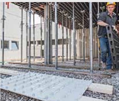
3. Installing the new formlining
